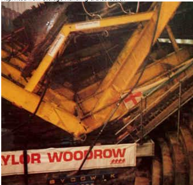
During the sliding operation
