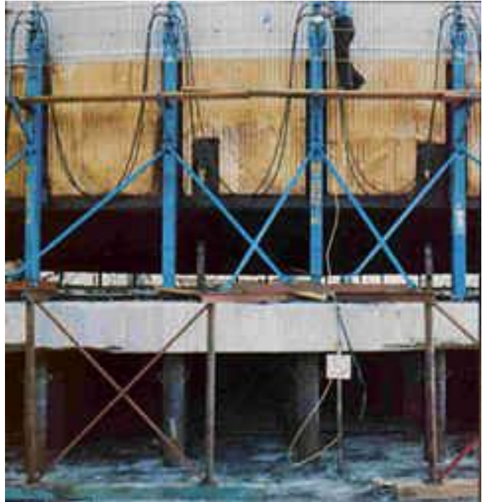
128x120 ft. Qatar. 720 tonnes. New base – New floor.
