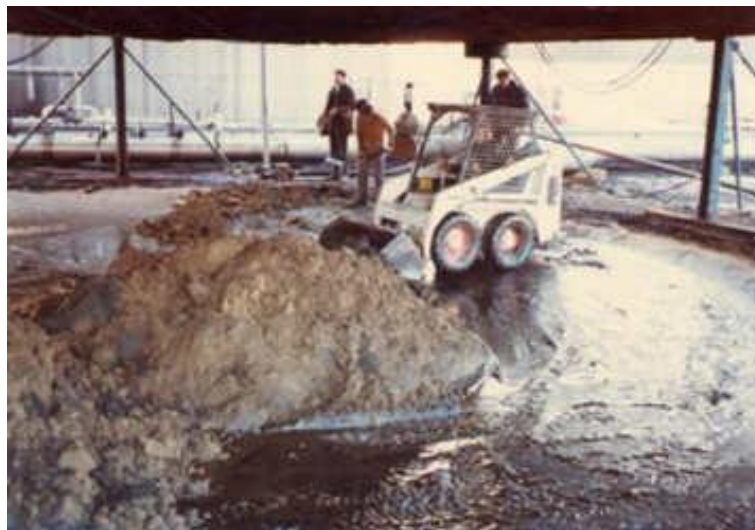
Base repair in progress
